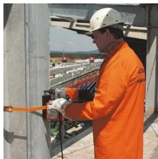
Shown in Action on Job Site
