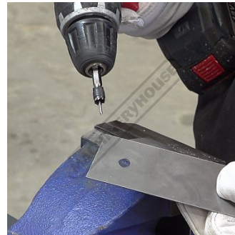
Spot Weld Removed & Top Plate Separated
